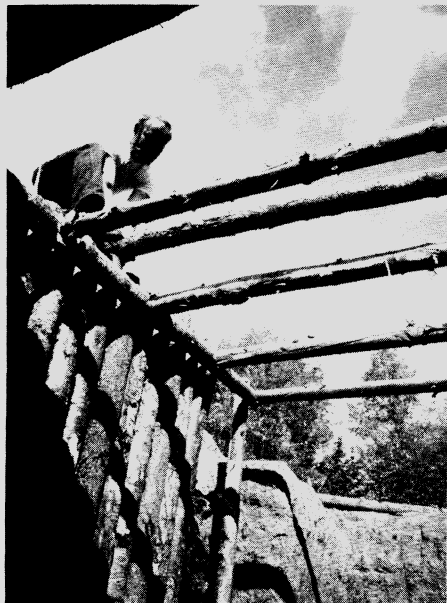
A father fits poles on an expedient blast shelter Photo © Krupp 1988
